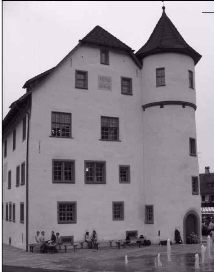
front view with restored sandstone reveals
