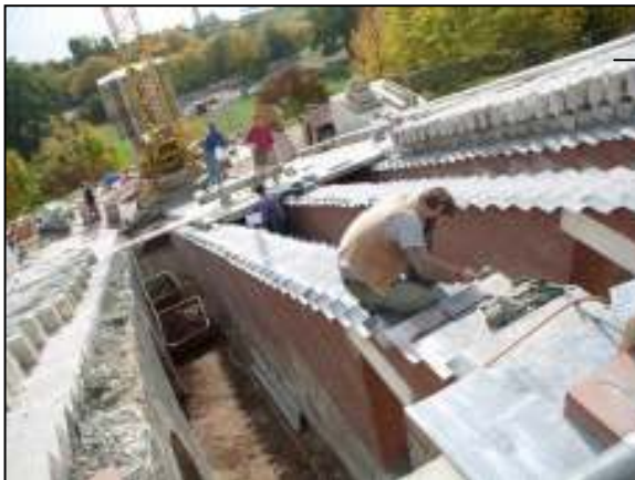
recreation of the substructure of the grand staircase
