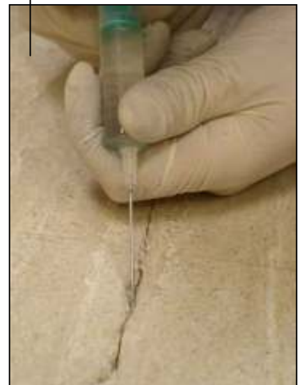
crack strengthening of the limestone
