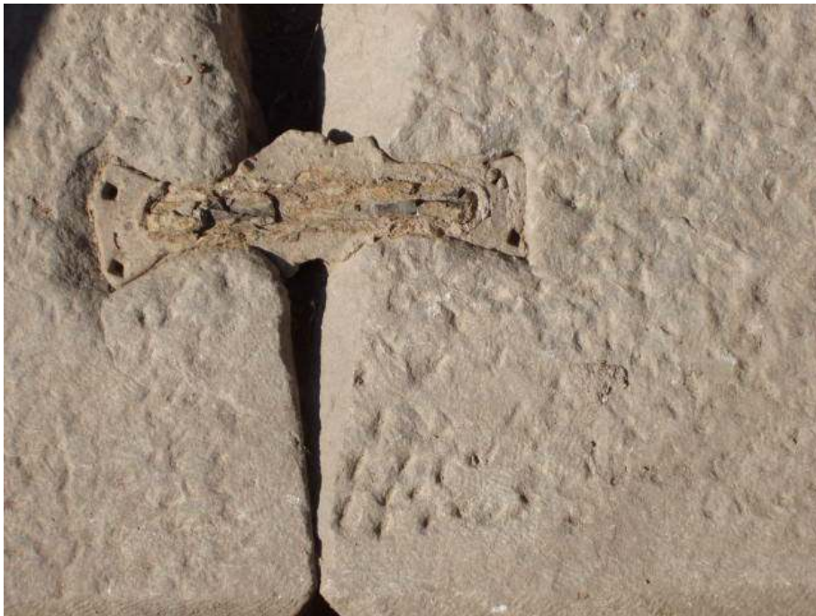
ancient dovetail clamp at the foundation of the market gate in miletus
