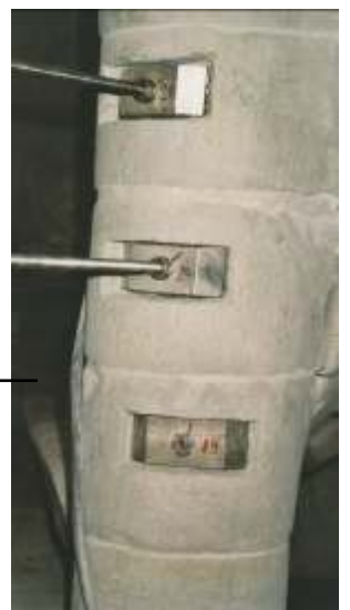
static securing of the spiral staircase during restoration
